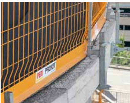
With the PERI Uni-Clamp and PERI Guardrail Post, the PROKIT Side Mesh Barrier can be used without drilling into the slab edge.
