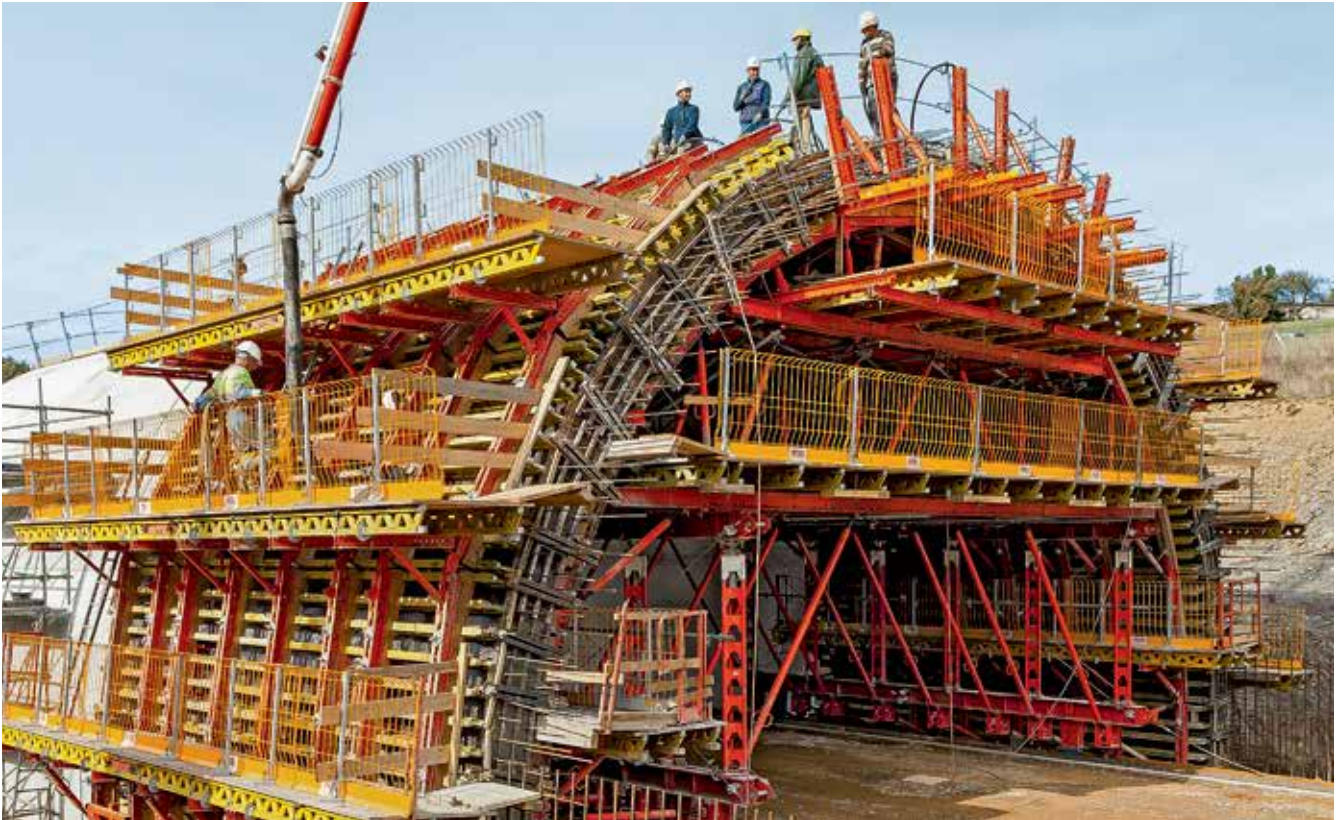
PROKIT EP 110 provides protection on the open edges of the working platforms of this tunnel formwork.
