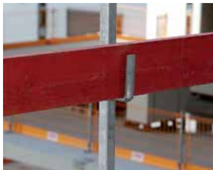
The holding brackets on the posts have nail and screw holes already in place so that handrail boards can be quickly fixed.
